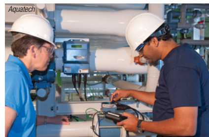
FIGURE 5. Aquatech's BioFilmPro is a sustainable data-driven solution that effectively controls biofouling by integrating real-time sensing and monitoring of biofilm formation with continuous electrochemical deactivation of bacteria and controlled biocide dosing
